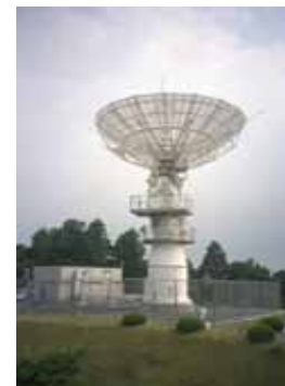
Masuda Tracking and Communication Station
