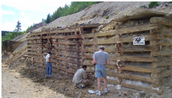
Figure 2. Wooden framework holding a spoil pile.
