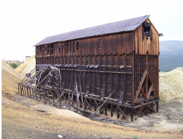
Figure 4. Old mill structure that sits above and protects sulfate accumulations.
