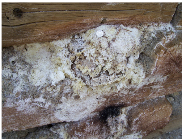
Figure 3. Sulfates precipitated from spoil pile.
