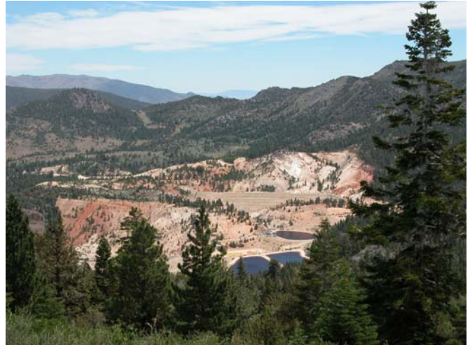
Figure 1: Field photo of the Leviathan mine site. Drainage from seasonal snows is channeled into a series of retaining ponds that are allowed to evaporate over the summer. Abundant iron oxide and alteration exposures are also present in the pit walls.
