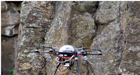
Figure 4: The Hexacopter equipped with a video camera captures images of the columns from a variety of altitudes.
