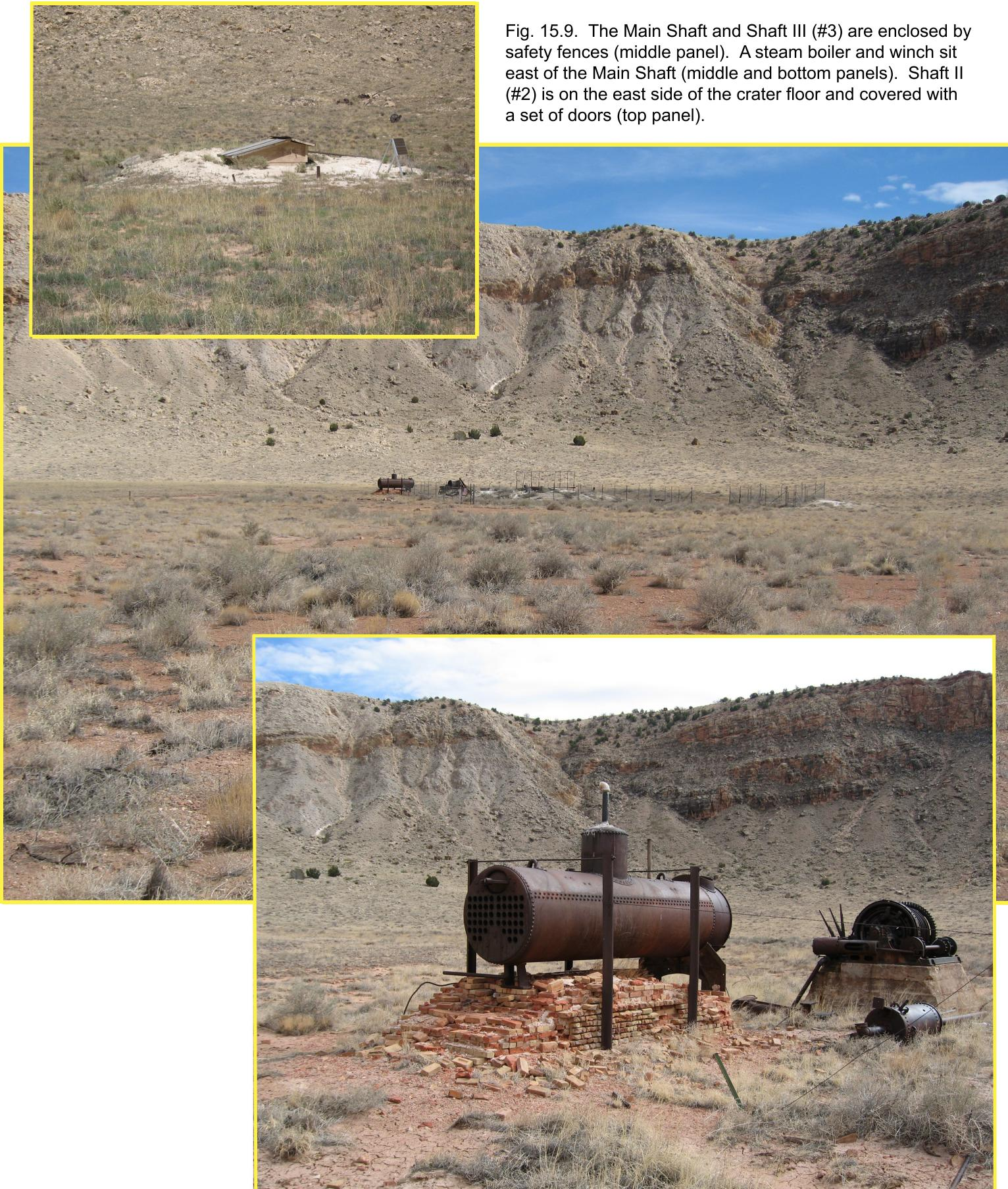
Fig. 15.9. The Main Shaft and Shaft III (#3) are enclosed by safety fences (middle panel). A steam boiler and winch sit east of the Main Shaft (middle and bottom panels). Shaft II (#2) is on the east side of the crater floor and covered with a set of doors (top panel).
